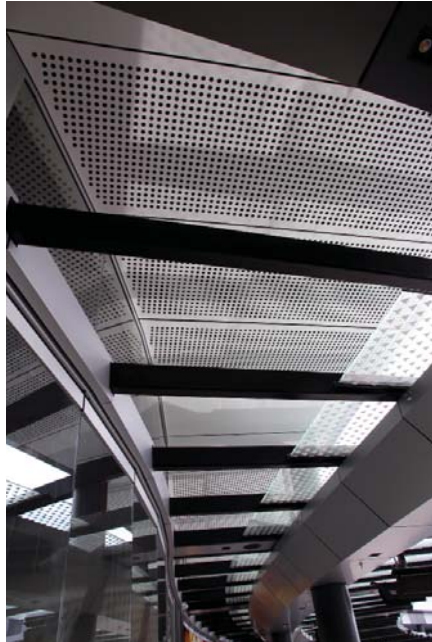
Perforated 9mm Fibre Cement - soffit panels custom shaped to follow curvature of external building
