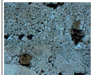
Poor quality concrete – Honeycombing and timber.
