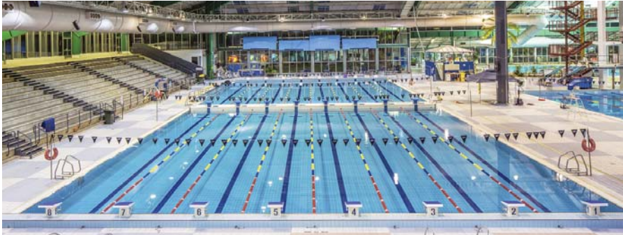
The Adelaide City Council together with the South Australian Government commenced refurbishment of the existing pools and areas with an estimated cost of $5 million
