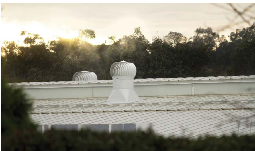
Rotary roof ventilators (whirlybirds) are an effective, environmentally-friendly solution
