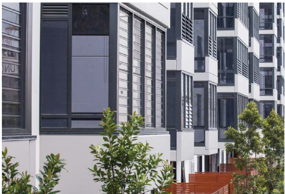
Safetyline Jalousie Louvre Windows installed in the apartment complex
