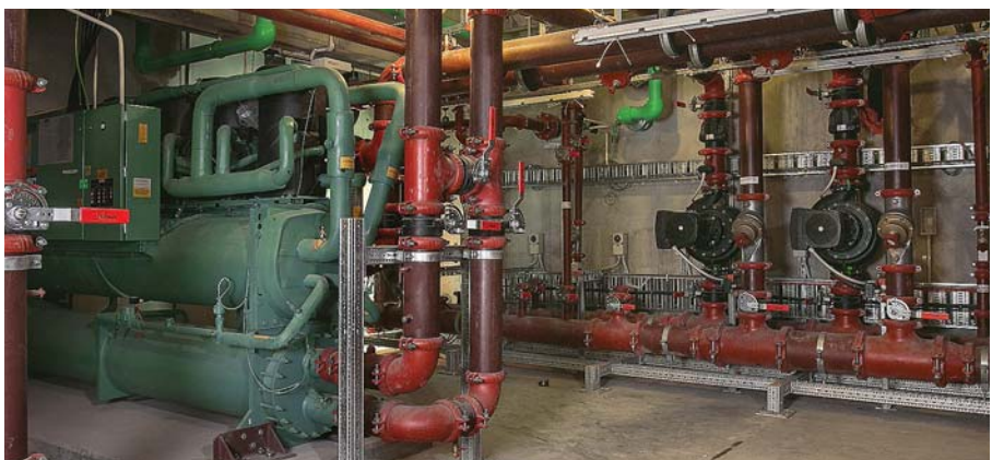
Library plant room utilising Victaulic products
