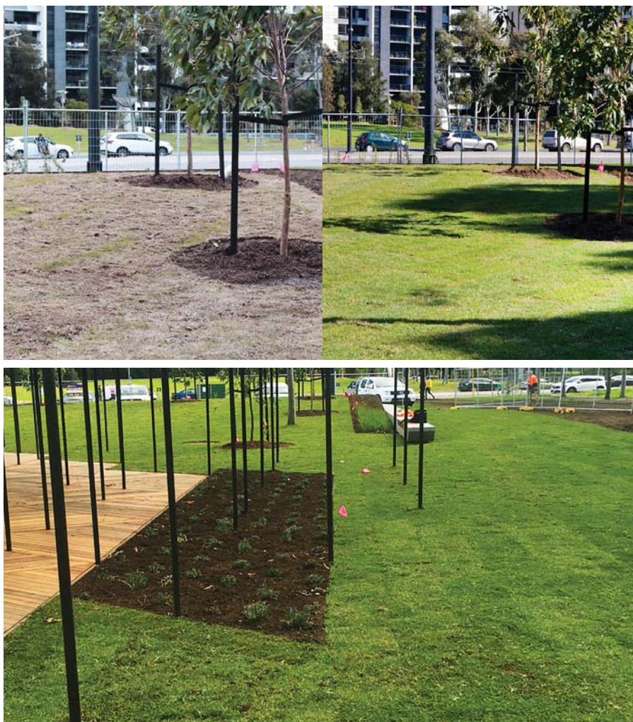
Top: Before and after replacing the inferior grass type with the specified Eureka Kikuyu Bottom: The turf installed at MPavilion at its new location in Melbourne's Docklands Park
