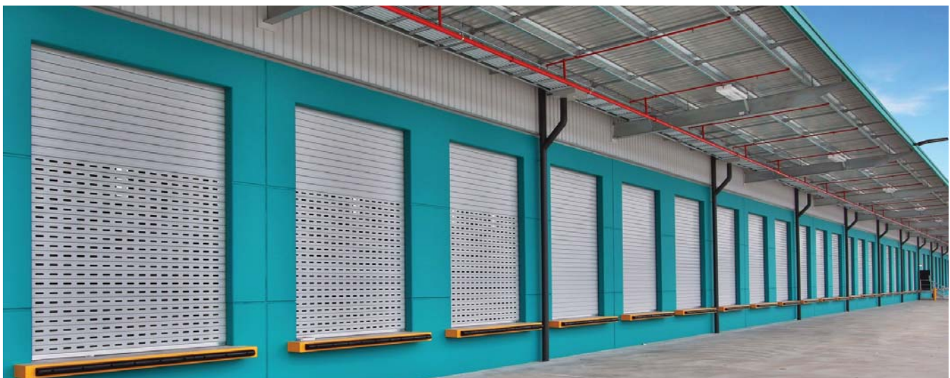
The Ezi-roll shutters installed at the facility and headquarters, at Tullamarine on behalf of Melbourne Airport and Toll Holdings Ltd.
