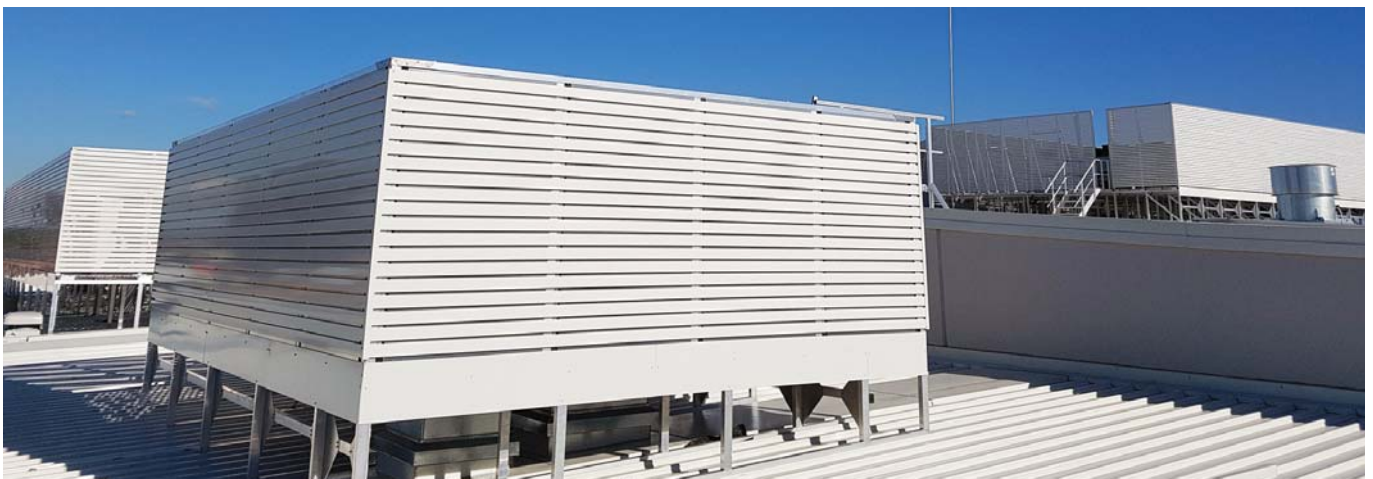
Con-form Series 3 raised platform system was installed to enclose the mechanical plant equipment in North Kellyville Square
