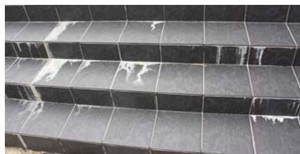
Efflorescence staining
