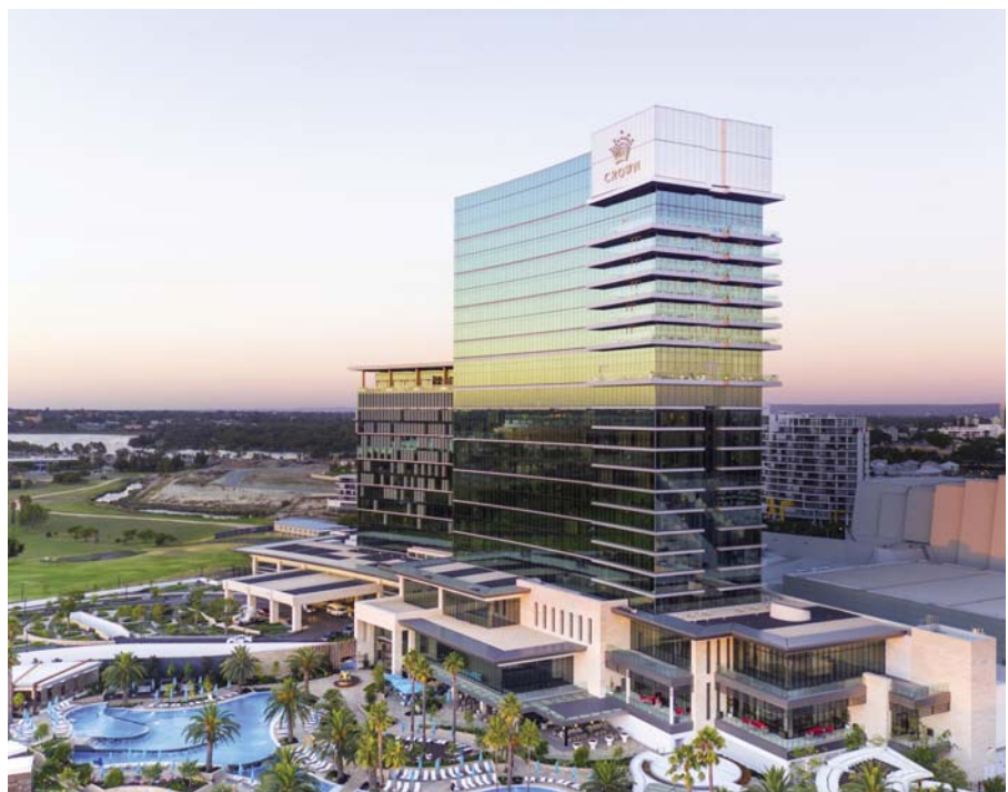
Views of Crown Towers in Perth, the expansion of which has marked it the first 6-star hotel in Western Australia
