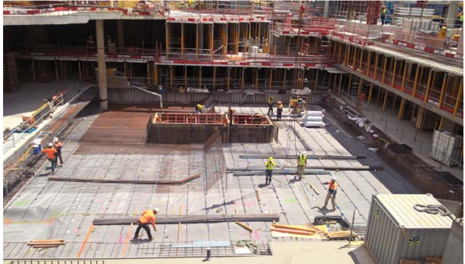
Works being completed at The Westin Perth, 480 Hay Street, Perth
