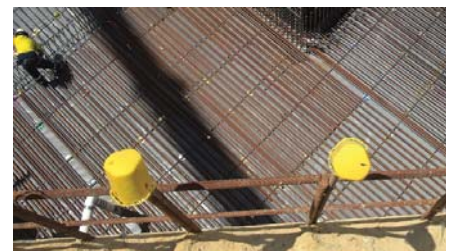
Top: Storing rolls of Proofex® Engage Bottom: Reinforcement over Proofex® Engage prior to concrete placement
