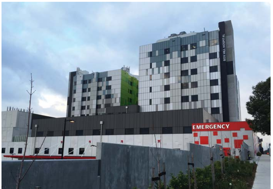
DEFLECTA ANTIMICROBIAL ® was applied at the time of pour, before carpet and vinyl installation, and meets the requirements of the Client under Bacterial Control Management and HAACP Food Safety
