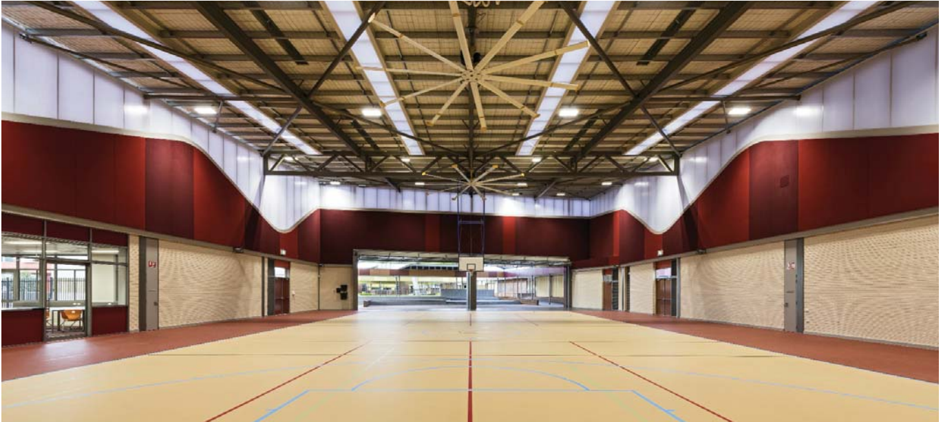
Inside the newly constructed Sports Hall, with Danpal rooflights and façade system, at Byford Secondary College
