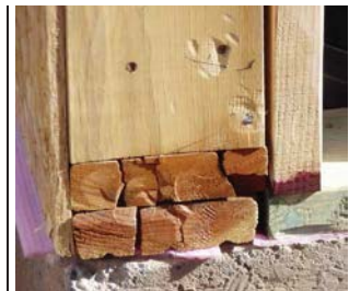
Poor quality timber construction – Split base-plate used.
