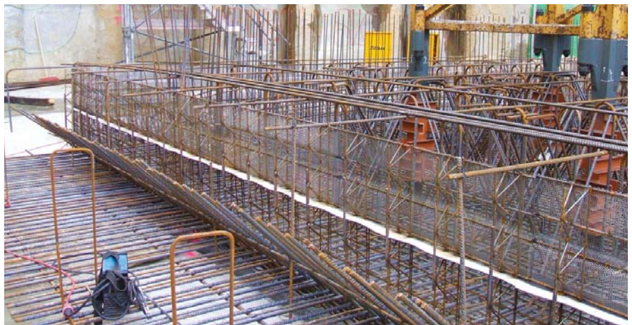
Stremaflex® formwork elements for the sealing of working joints on site of construction
