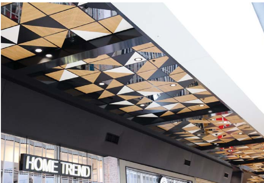
Custom feature Triangular ceiling manufactured in Laminex laminated material – solid and perforated panels
