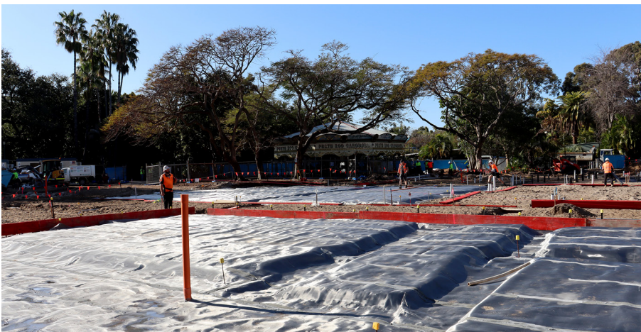
Termimesh sheets installed above the damp proof membrane of the new Function Centre
