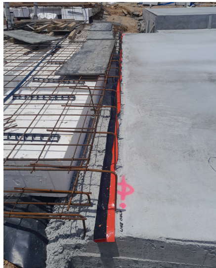
Kordon system installation for cold joint protection to adjoining slabs pre pour
