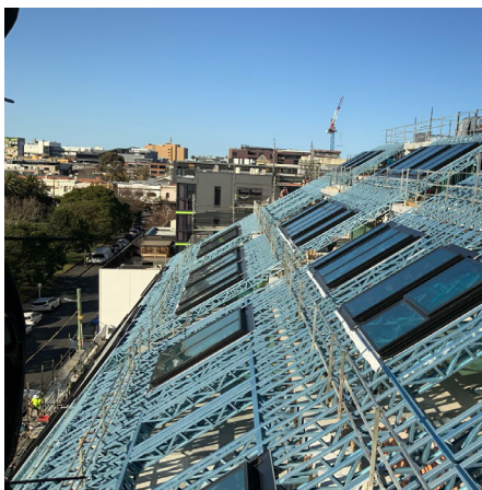
The sloping facade structure is a TRUECORE® steel frame engineered to support the tiles as well as the distinctively large windows
