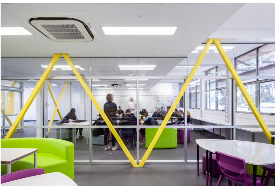
Internal view – the exposed earthquake bracing
