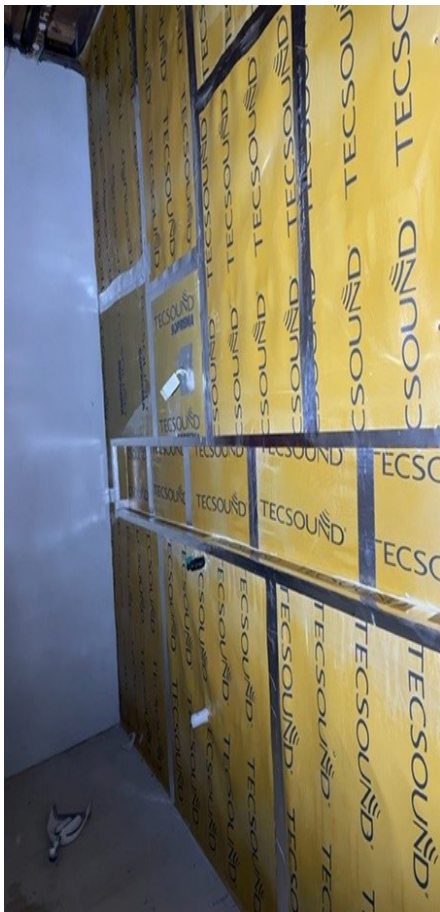
TecSound SY installed between studs preventing sound transmission
