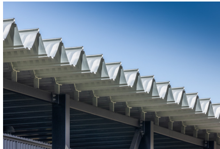
ARAMAX® roofing was specified with an unpainted ZINCALUME® steel finish
