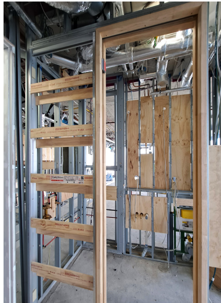
CS MidWay Cavity Slider with grooved jambs, ready for installation
