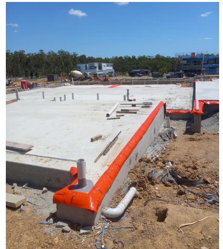
Kordon system perimeter installation prior to frames being erected
