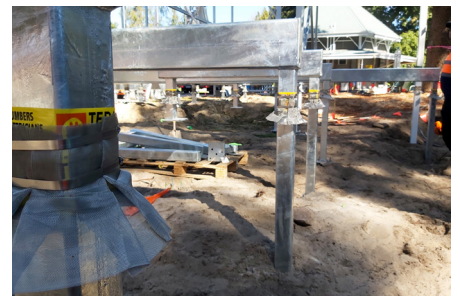
Termimesh termite mesh caps installed around the top of columns supporting the new Visitor Café
