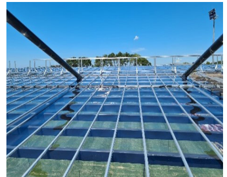
Engineered Step Joint supporting 10.5-meter sheets
