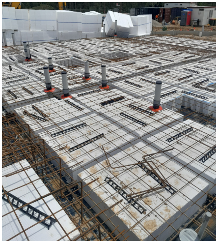
Kordon system installation to service penetrations to a waffle pod slab pre pour
