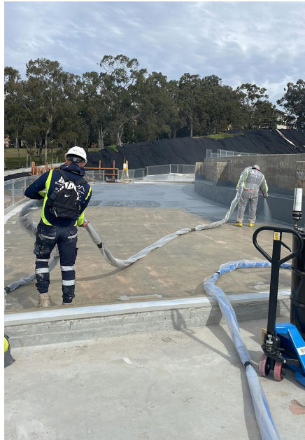
Spray application of Polyurea WHE110
