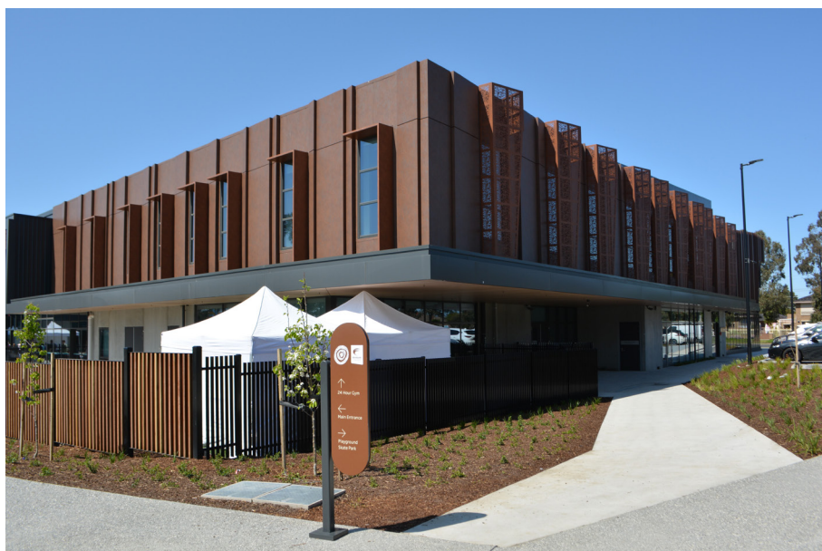
The Askin Vivid Insulated Panel & Aluminium façade system in custom colour matched Weathered Iron
