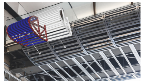
Custom designed and Prefabricated lightweight steel panels
