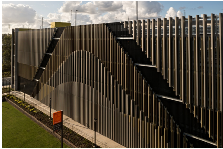
Lightweight PERMALITE® aluminium purlins create a vertical vein façade
