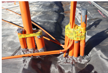
Termiflange termite mesh collars installed around clustered vertical slab penetrations
