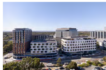
Murdoch Square mixed-use development situated in the south of Perth's CBD
