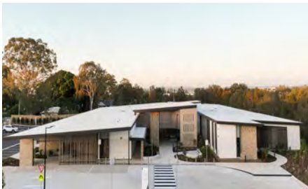
Completed Redlands Satellite Hospital with Termimesh System installed - Image supplied by Hutchison Builders
