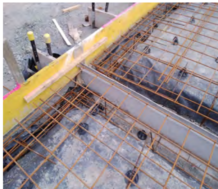
Pre-installation of Termimesh along a construction joint before concrete slab pour
