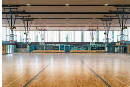
The inside view of the Baldivis Indoor Sports Complex, which displays Danpal Façade Systems and also gives the view of the natural surroundings
