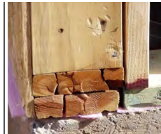
Poor quality timber construction – Split base-plate used.
