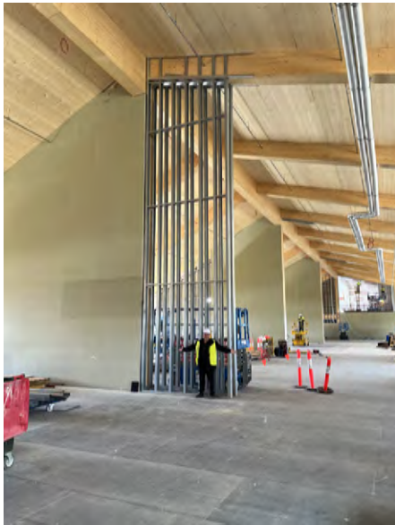
10.8-meter-high internal steel wall framing
