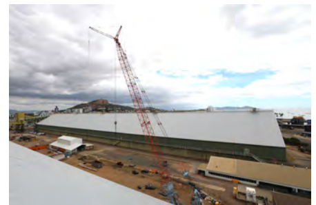
Townsville Bulk Sugar Terminal construction
