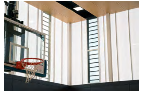
A closer view of the Danpal Polycarbonate façade systems integrating with a series of glazed louvres that provide both natural lighting and ventilation
