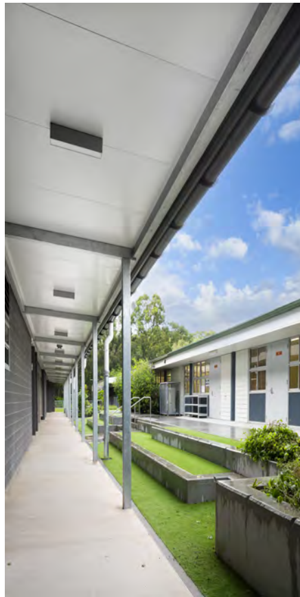
Underside of External Connecting Walkway
