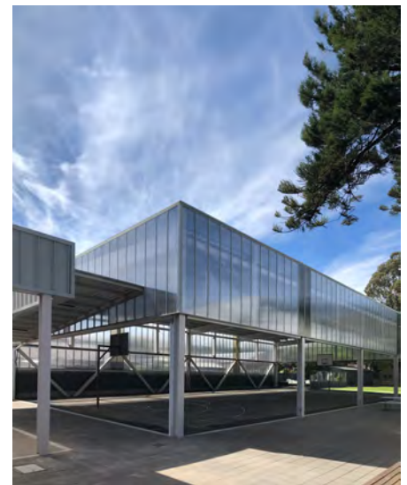
SUNLITE 10mm Twinwall Polycarbonate Facade
