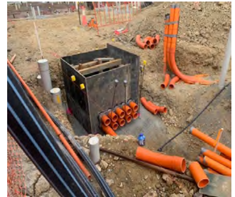
Vertical installation of Termiflange termite mesh collars on horizontal penetrations in an electrical pit
