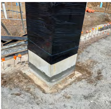
Construction joint protection around pre-formed square pier
