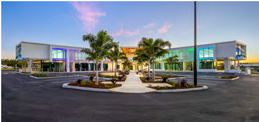
Compliance reached with Tactile Systems installed on the kerb ramp at dusk
