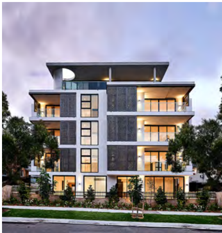
Exterior view of apartment block
