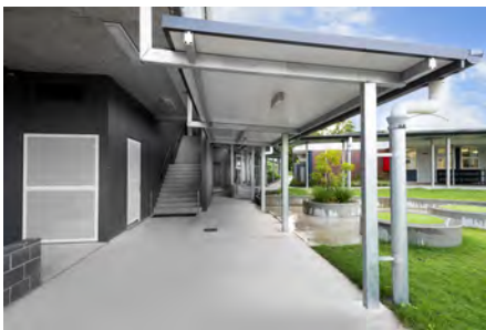
External Connecting Walkway with HDG Structural Steel
