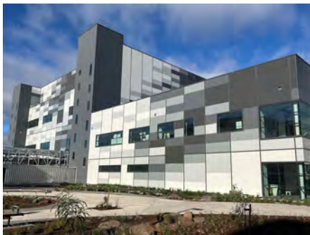
Volcore Vivid External Facade
