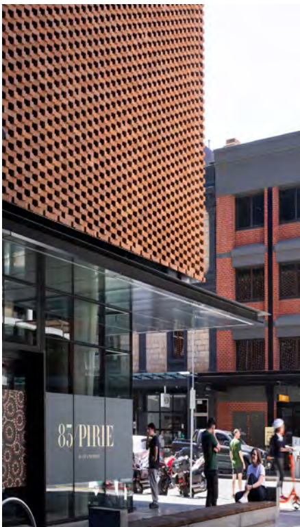
83 Pirie St completed façade
