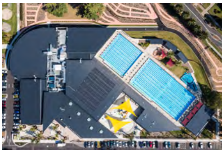
Aerial drone image of the whole site, showcasing the vast number of panels used on the roof
