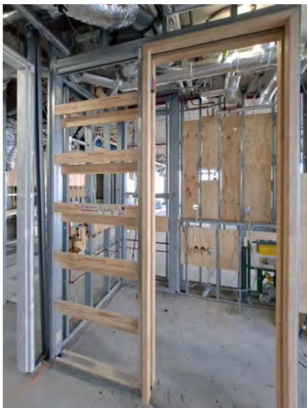
CS Cavity Slider ready for installation
