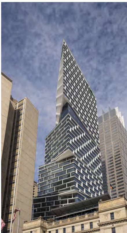
Cantilevered, twisting glass villages maximise views and reduce heat
