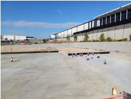
Pre-installed Kordon Kollars to penetrations to a pre-poured concrete slab
