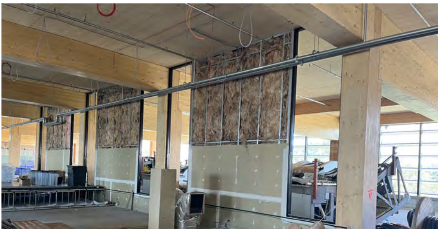
Steel studs integrating with mass timber and glass
