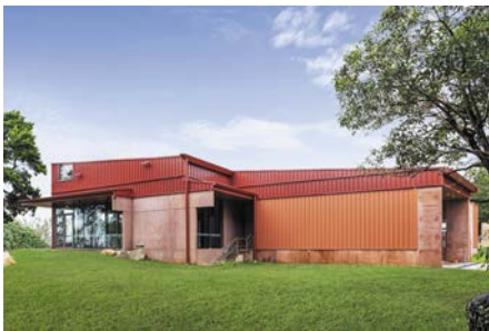
Stratco Hiland Tray cladding in COLORBOND® Fire Opal and Clay Brown contribute to the striking colour pallet of QUAMPI Arts & Cultural Centre
