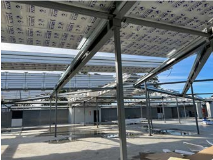
Beginning of installation
