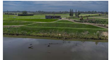
Completed reconstruction and turf installation on riverbank
