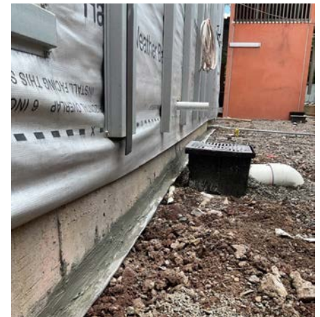
Termshield Installation isolating a construction joint at the perimeter pre external pathway concrete pour
