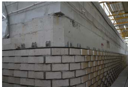
Leviat Ancon MDC provides seamless support for curved corners
