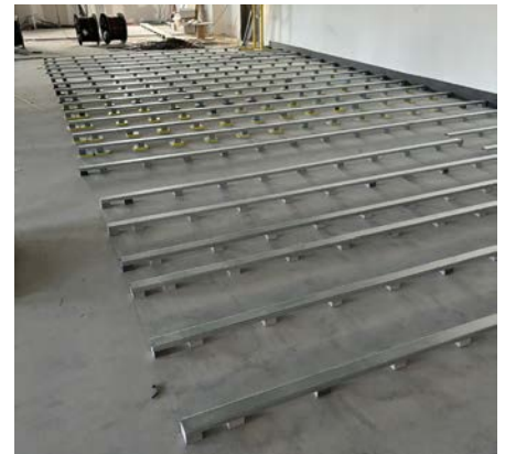
Construction phase - PUR isolation blocks and channels installation
