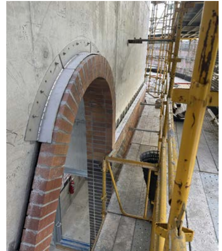
A distinctive brick arch had bespoke hanging plates for soffit bricks beneath
