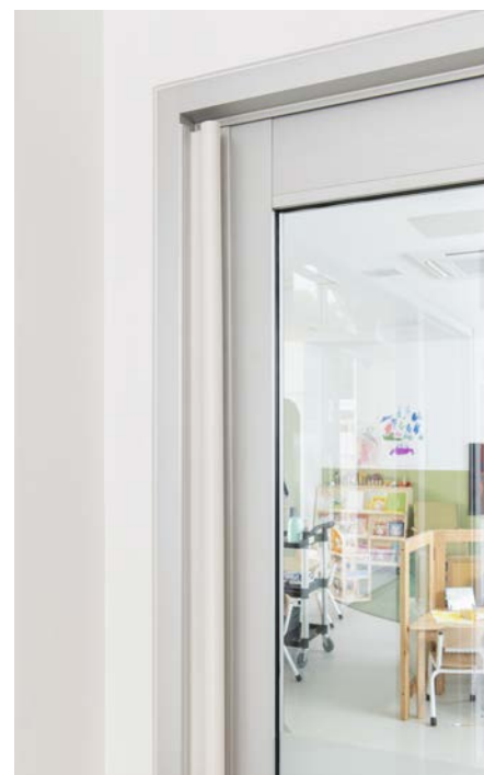
Raven finger guard seals provide protection from finger-pinch injuries in the doors in the Beyond early learning centre
