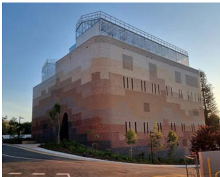
UQ's Plant Growth Building makes up part of the Plant Futures Facility
