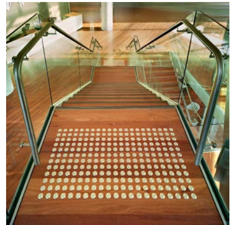
Main staircase – nosing and tactiles
