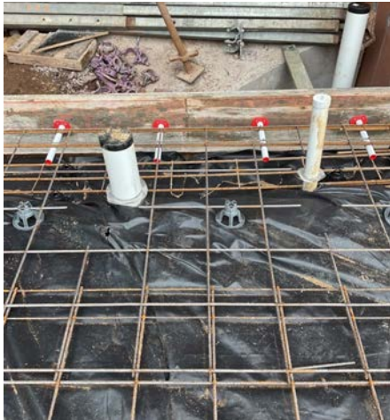
Termshield Installation of slab penetration flanges pre concrete pour
