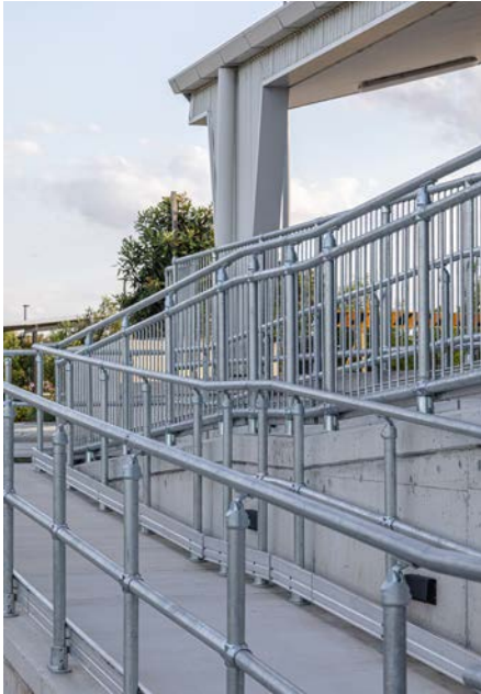
Accessible ramp with Assistrail handrails at South Pine Sports Complex, providing easy entry to the seating area
