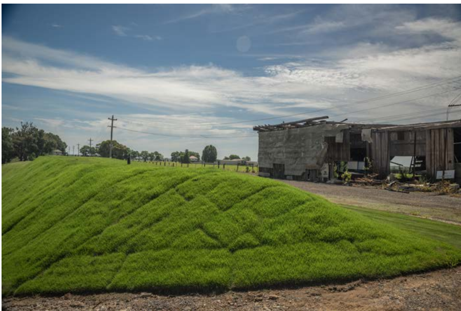
Recently installed turf grass for soil stabilisation
