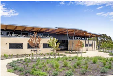
Breezway Powerlouvre System installed in the Clifton Springs Primary School
