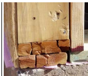
Poor quality timber construction – Split base-plate used.
