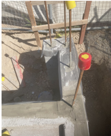
Termshield installation Isolating an engaged pier at top of slab height
