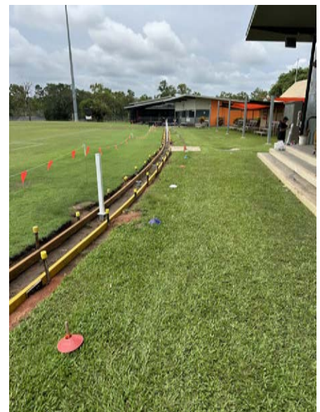
Installation of Headingly Picket Fence DXC Arena Darwin
