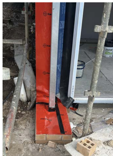
The above image illustrates Kordon's application on a brick pier, where it wraps around and seals a steel column before integrating into the perimeter barrier. Left untreated, such a pier could provide a concealed entry point for termites, making expert installation crucial.
