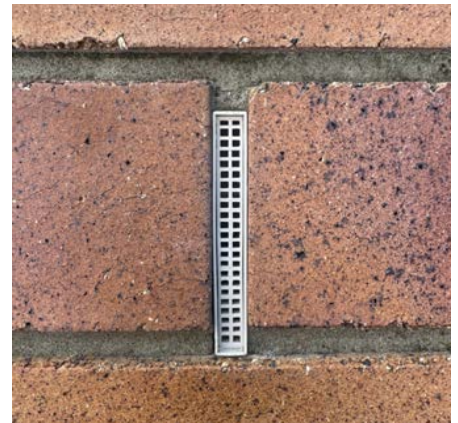
70mm Bushfire Weepa in brick wall
