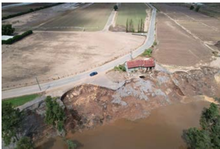
Riverbank destruction after flooding
