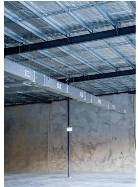
Wide shot of the retail precinct interior, highlighting the clean lines and minimal joints of the installed ductboard system
