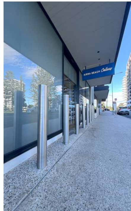
Stainless Steel Bollards
