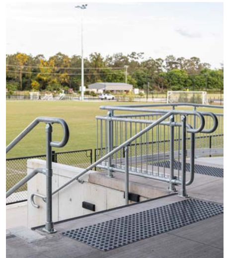
Staircase and ramp leading to the sports field at South Pine Sports Complex
