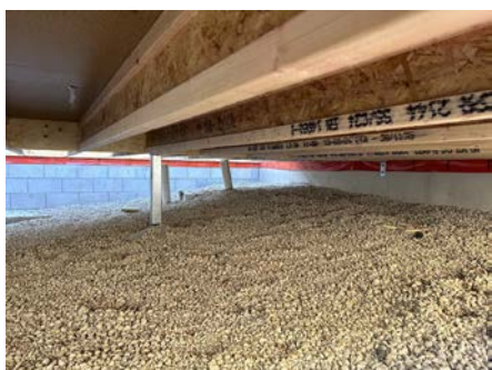
The Kordon installation behind a timber pole plate positioned against a block wall, extending to the concrete slab. This setup ensures the pole plate compresses the barrier against the slab, effectively blocking termites.
