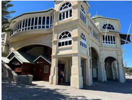
The window frames were coated with Taubmans 3 in 1 prep undercoat, and All Weather semi-gloss
