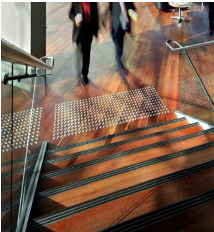
Stair nosing and tactiles
