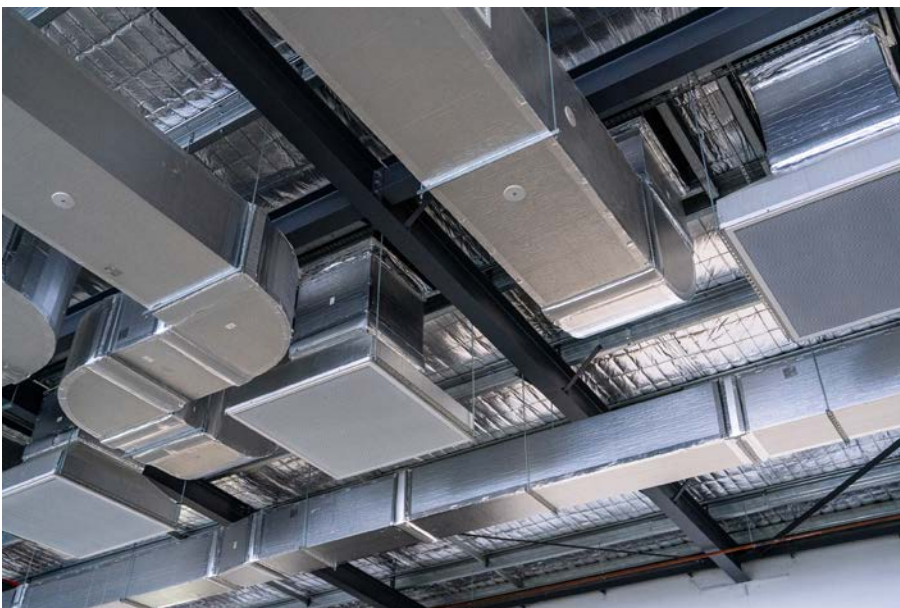
Close-up view of the exposed Kingspan ductboard system, showcasing precision fabrication and seamless integration with the open ceiling design for improved energy performance and aesthetics
