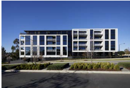
The façade features a framing pattern with contrasting materials including warm grey brickwork and vertical metal balustrades
