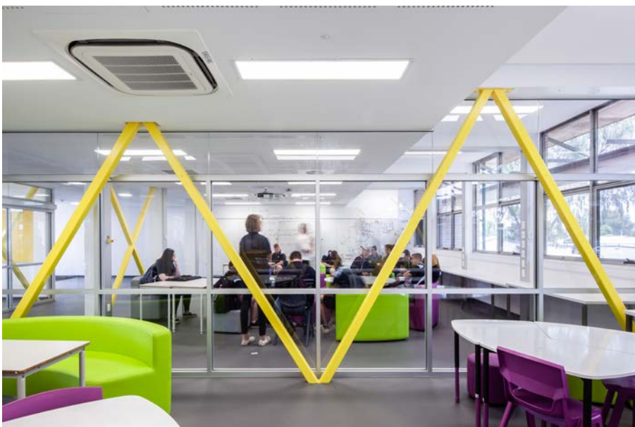
Internal view – the exposed earthquake bracing
