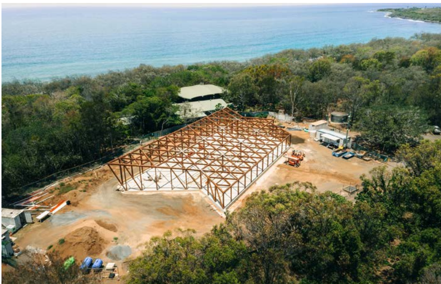
External diagrid structure (Hyne)
