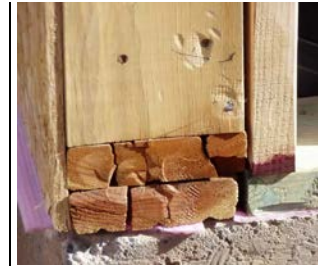
Poor quality timber construction – Split base-plate used.
