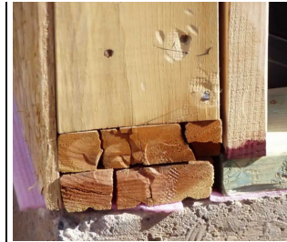
Poor quality timber construction – Split base-plate used.
