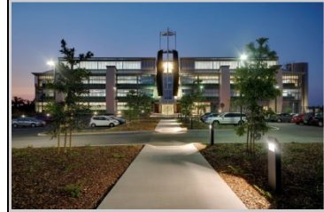
Dandiiri Contact Centre, Zillmere, Brisbane – achieved 6 Star Green Star – Office Design V2 in 2010.
